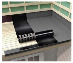
As a general rule, a joint-sealed roofing may on renovation sites be installed on top of the old even bitumen roofing, if the structure ventilation is working and the underlaying structures are in order. The new roofing must be installed in parallel with the old roofing so that the longitudinal seams of the roofings do not fall in the same place. Any bumps/pouches must be cut as well as glued and nailed to the underlay before the new roofing is installed.
