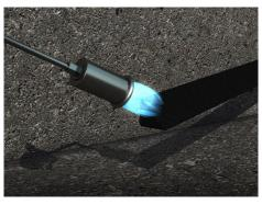
Heat the connecting surfaces of the bitumen triangle fillet end with a gas flame, and press end into place immediately.
