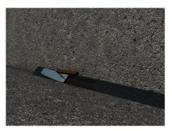
Ensure the adhesion of the bitumen triangle fillet to the base with a trowel or roller, for example.
