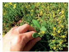
Any unwanted plants, tree seedlings and extra material such as leaves and needles are removed from the roof. A thick layer of leaves or needles on a sedum roof may cause severe damage to the sedum.
