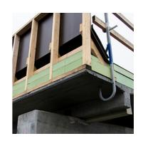
Kerabit 5000 TOP FR has a reinforced polyester felt as a carrier. The bottom surface of the product features modified torch-on bitumen, and the top surface slate granules.
